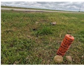
**Photo #8** Culvert and typical view of tile drain inlet.
