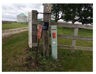
**Photo #6** AT&T underground cable marker – AOI 1.
